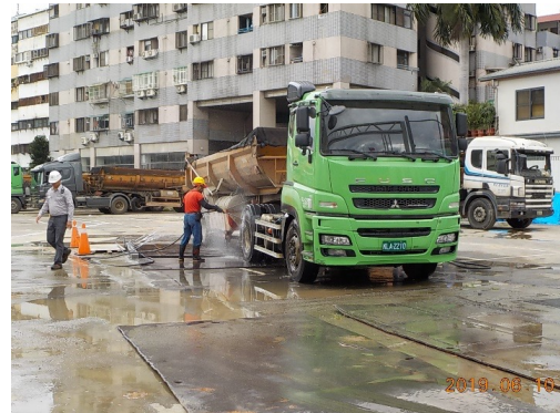
The wash platform uses a high-pressure washer to wash the tires and body of vehicles as they exit.
